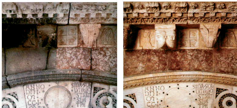
Figure 5: Foligno Cathedral; limestones, marbles and travertine – before and after restoration (Courtesy of B. Moroni and G. Poli, Perugia).
